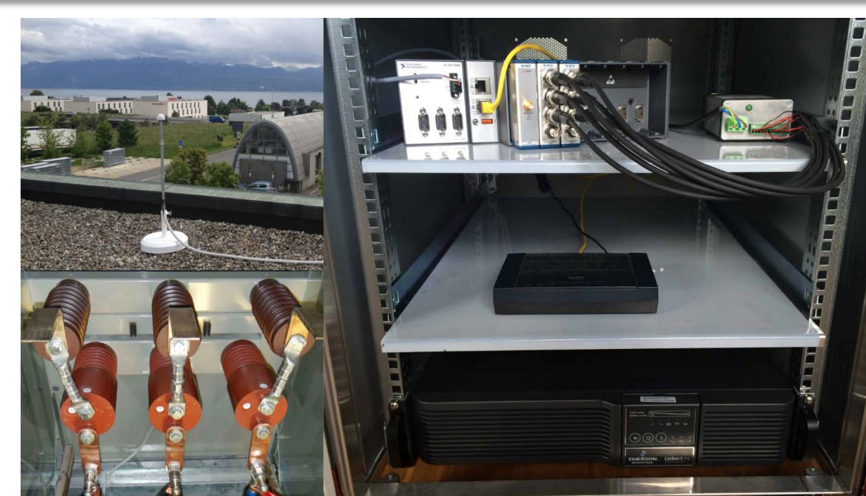
Typical setup installed in the substation: GPS antenna, sensors, PMU device with modem and UPS.
